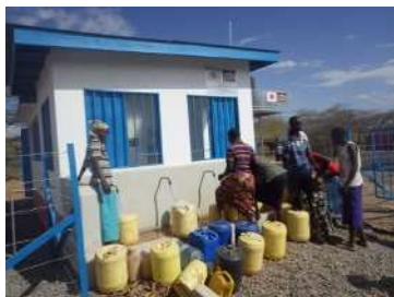
ケニア国大バリゴ県村落給水計画 The Project for Rural Water Supply in Baringo County (Kenya)
