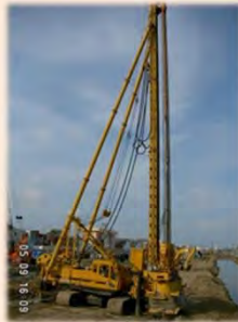
Deep soil mixing work along canal (overseas project)
