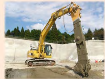
Mass-stabilization work for facilities of factory
