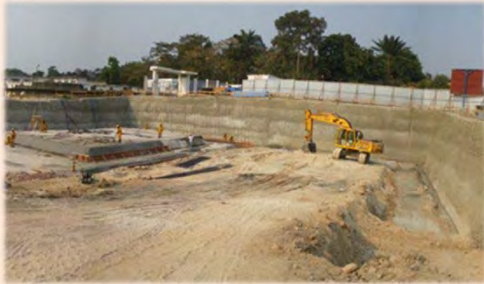
Retaining wall by Soil Nailing combined with shot-crete (overseas project)
