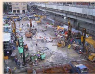
Chemical Grout as ground protection for tunneling work (overseas project)
