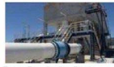
Tugun Desalination Plant
